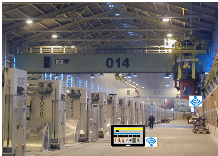
Figure 3. HMI screen on tablet.
